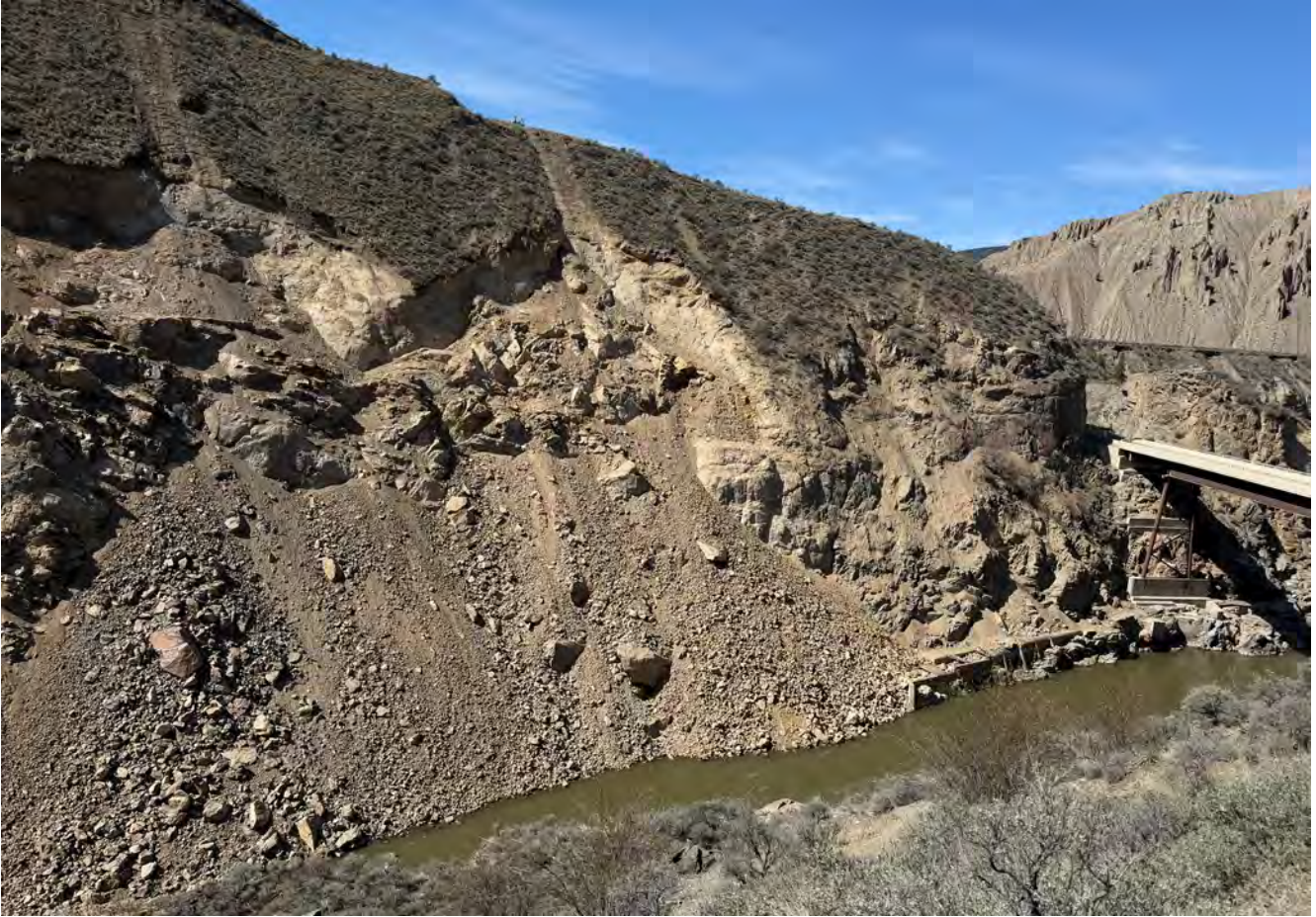
Farwell Canyon Tension Crack Area, post slope stabilization work.
